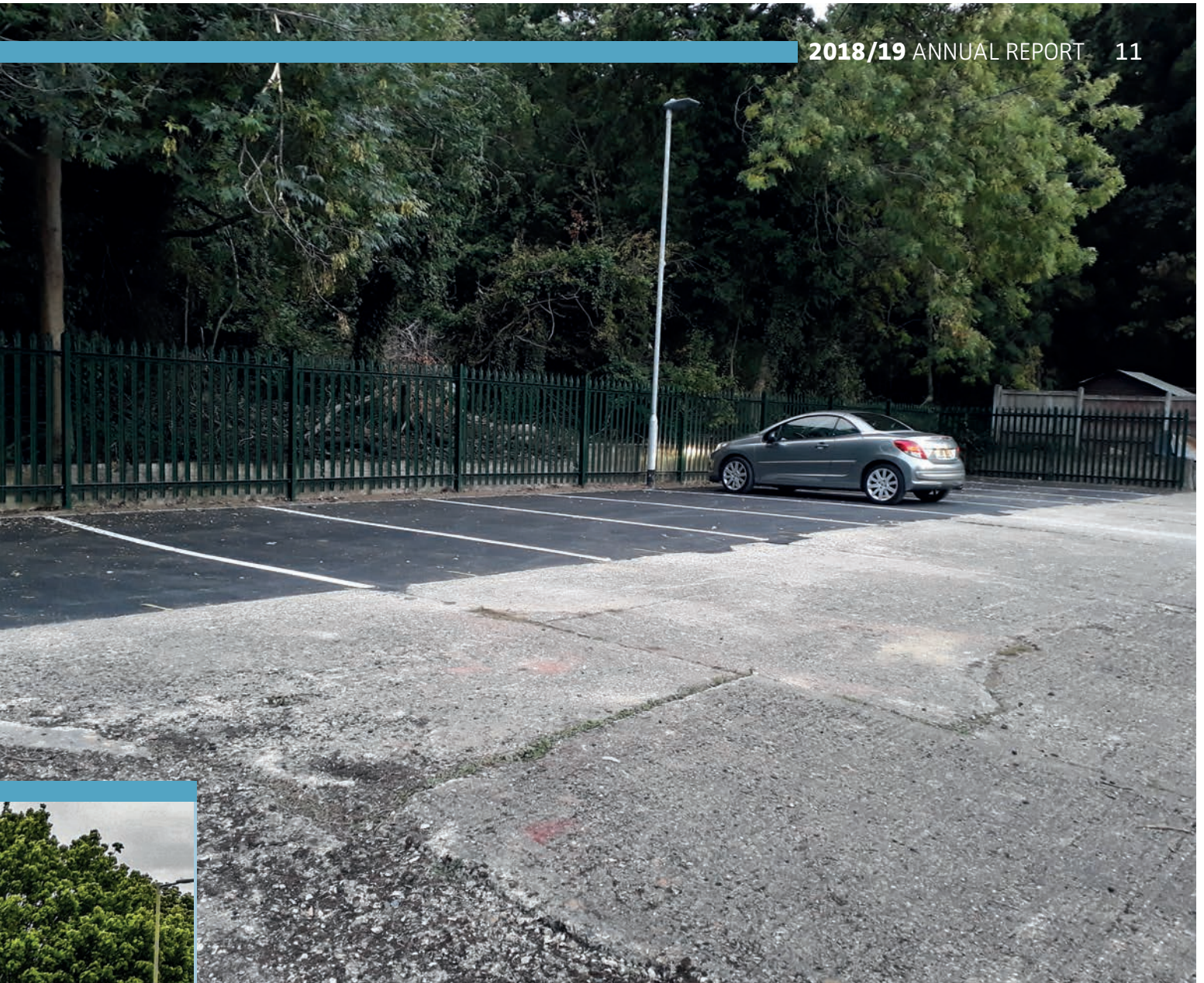
Great Dell, former garages site
